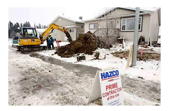
Capital Excavating Ltd. works to disconnect the water and sewer lines on one of three homes in Calmar that are to be demolished by Imperial Oil.
